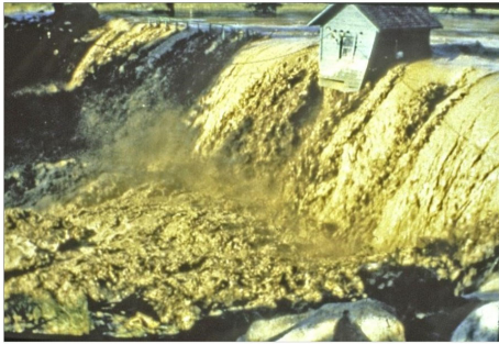
Cascade Dam overtopping. The dam was a 17-foot-high gravity concrete dam (Photo source: G. D. George from USGS files).
