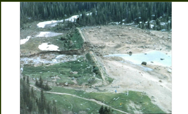
Lawn Lake Dam Breach morning of failure July 15, 1982 (Photo source: the United States Bureau of Reclamation).
